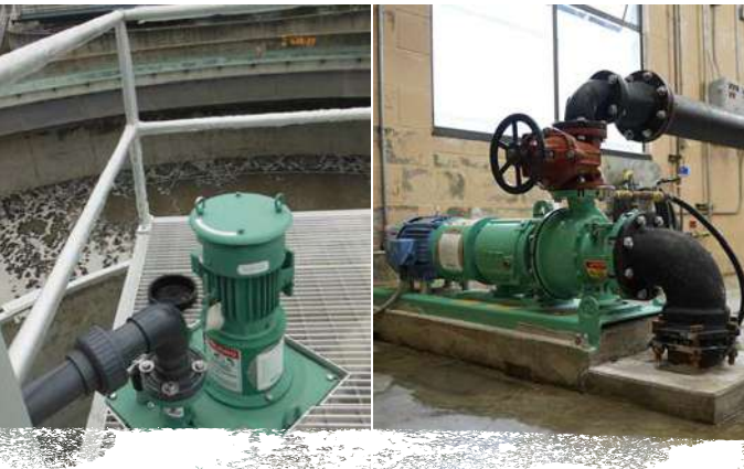
Primary Clarifier Scum
